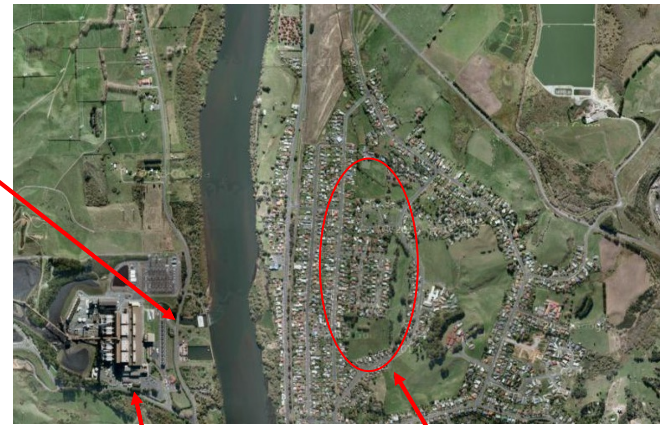
Coal-fired power station.
