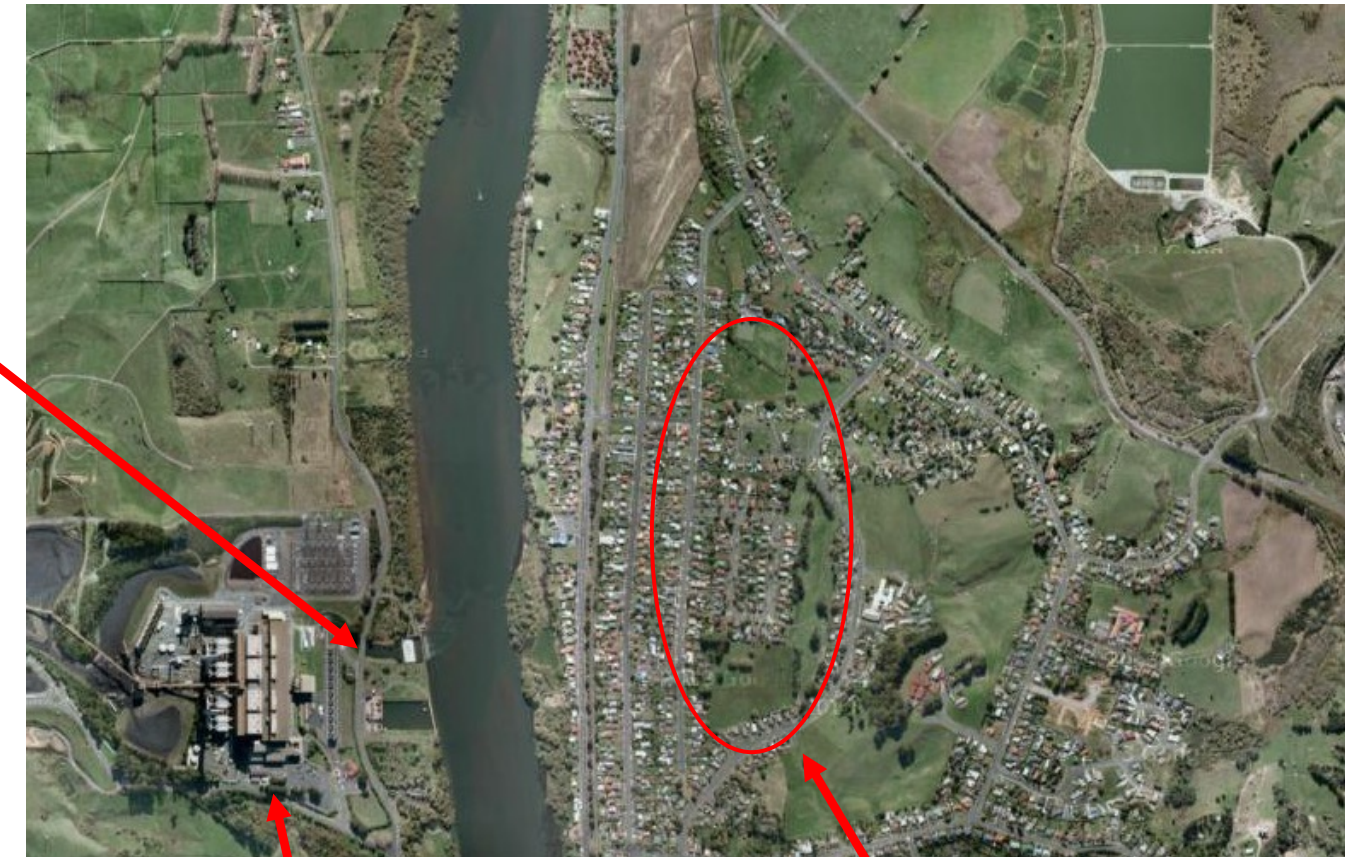
Coal-fired power station.
